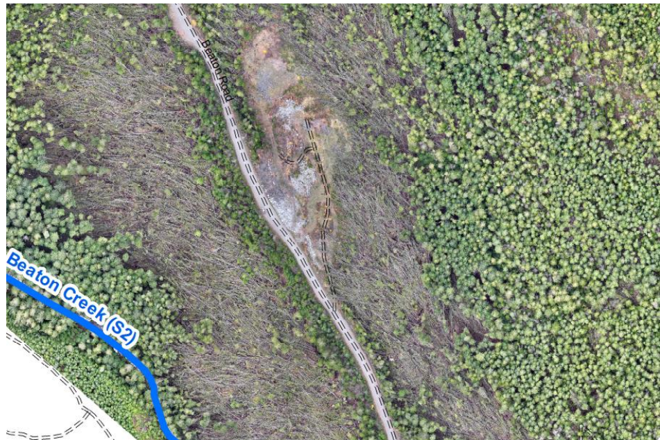
Drone plan view of catastrophic windstorm damage
