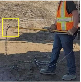
Position the pole hook onto the second link b) from the collar of one of the wrapper ends
