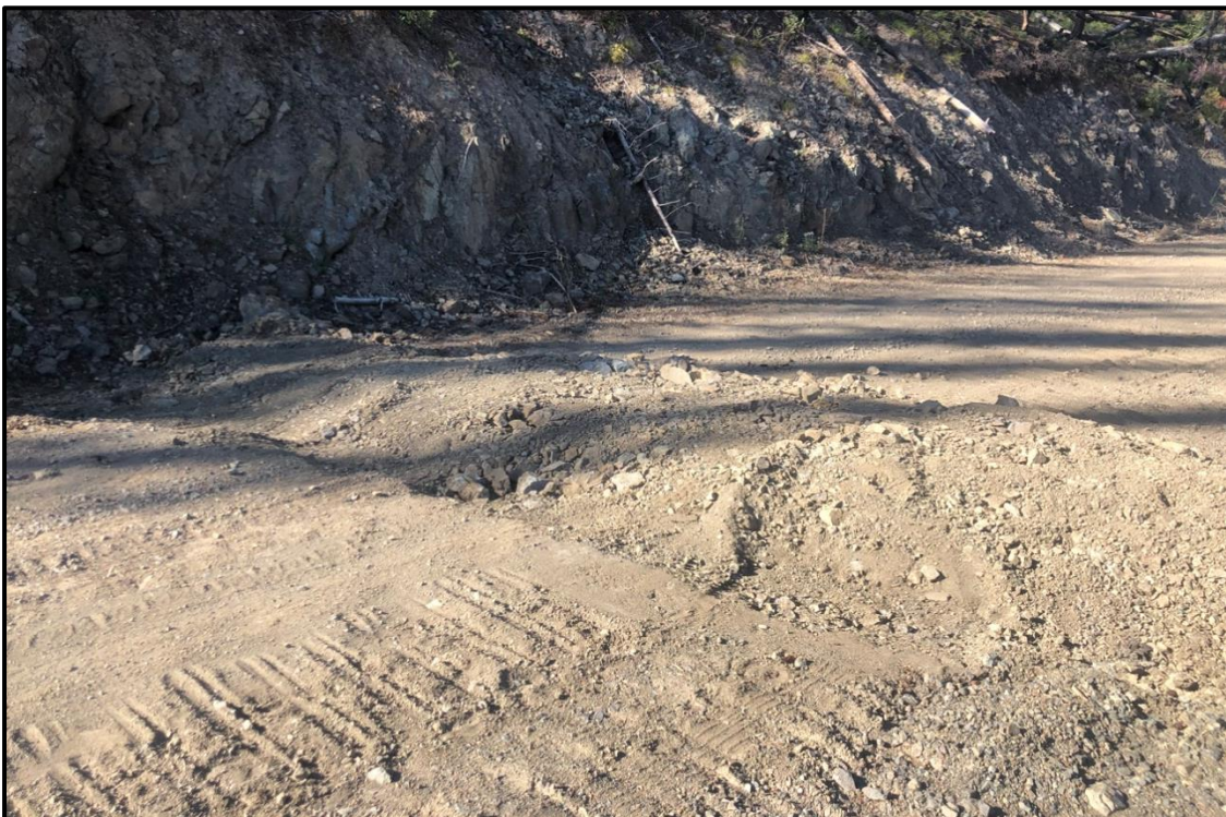
Images of water bars on a deactivated resource road
