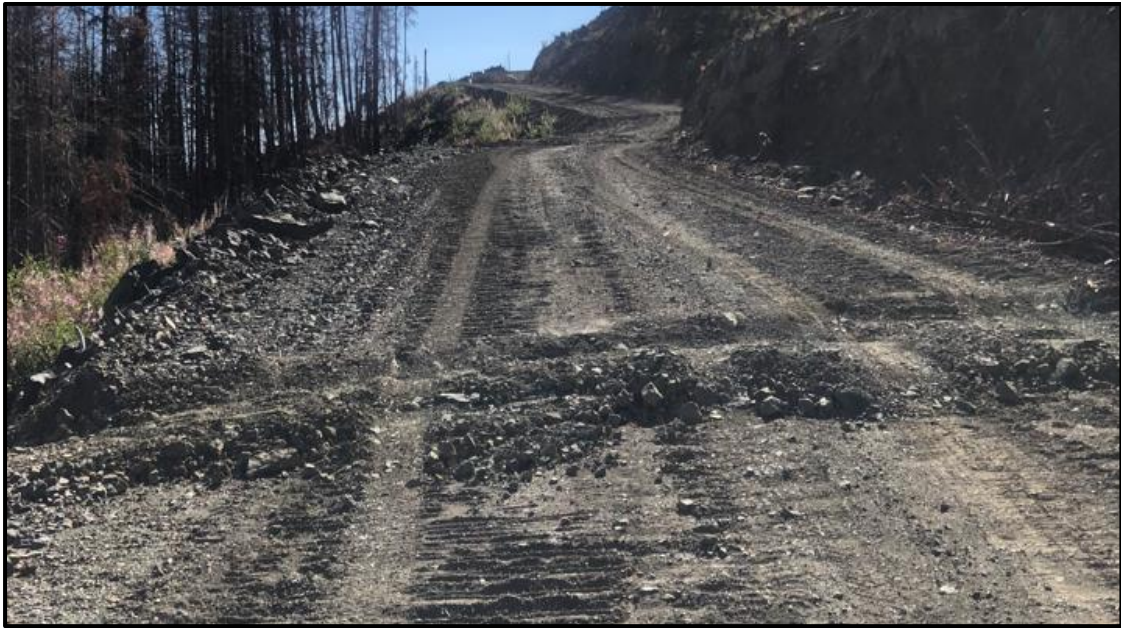
Images of water bars on a deactivated resource road
