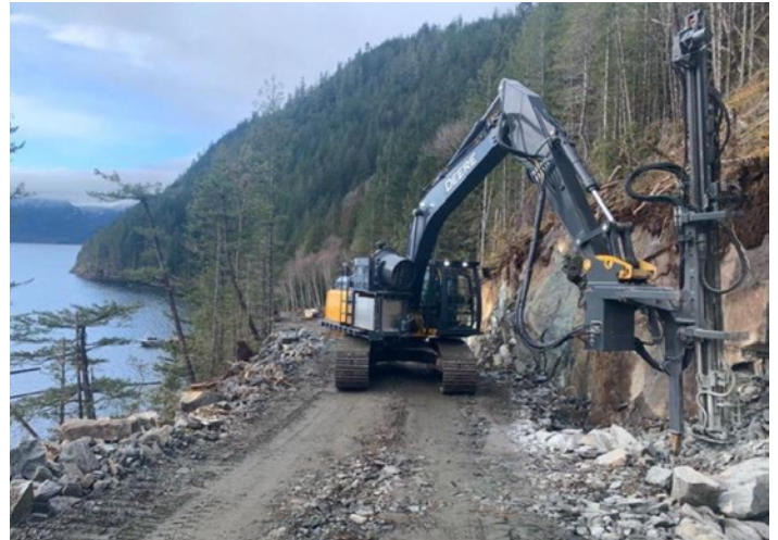
Photo Credit: Mark Ponting – Ponting Contracting
