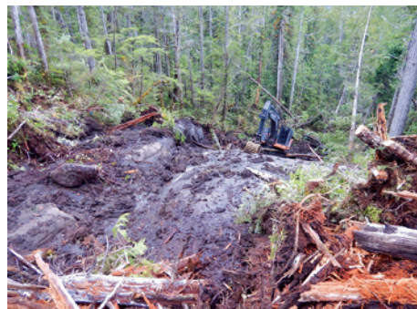
Excavator in a construction initiated slide.
