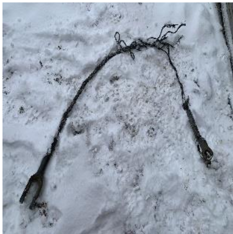
Emergency cable failure after cab free-fall
