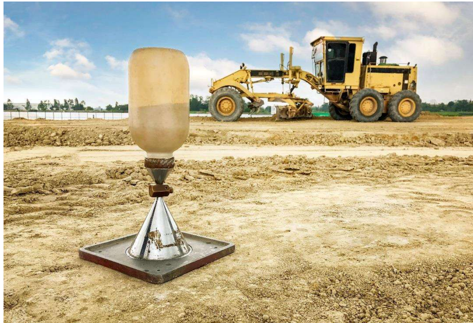
Example of a sand cone test set up
