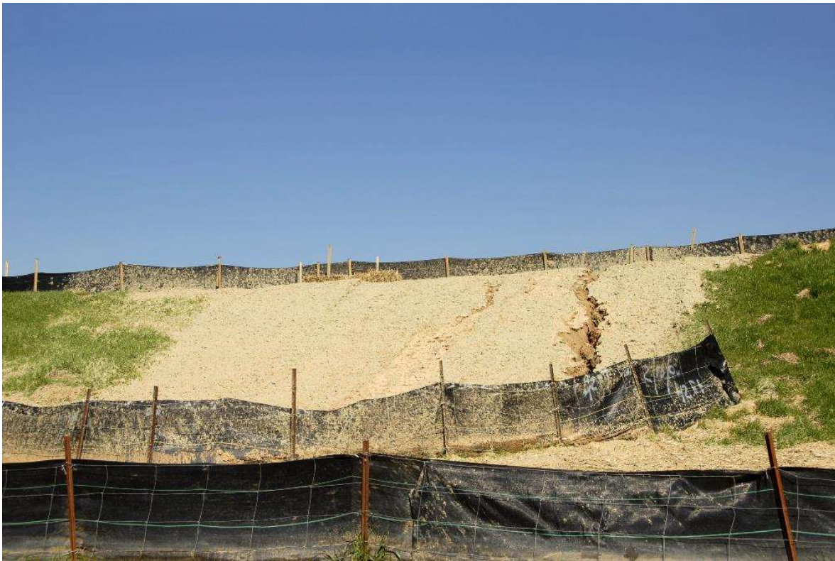
Use of silt fences and grass seeding to control erosion
