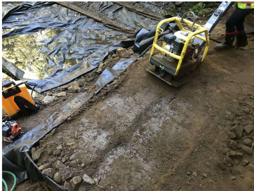
Plate compactor, picture from Chris Cole, P. Eng.
