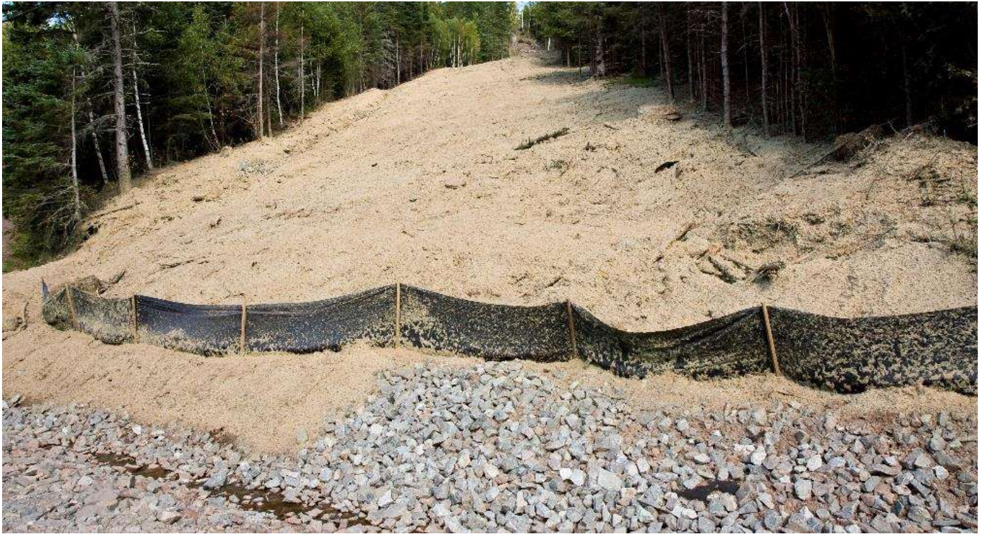
Grass seed, silt fencing and rock armouring used to control sediment
