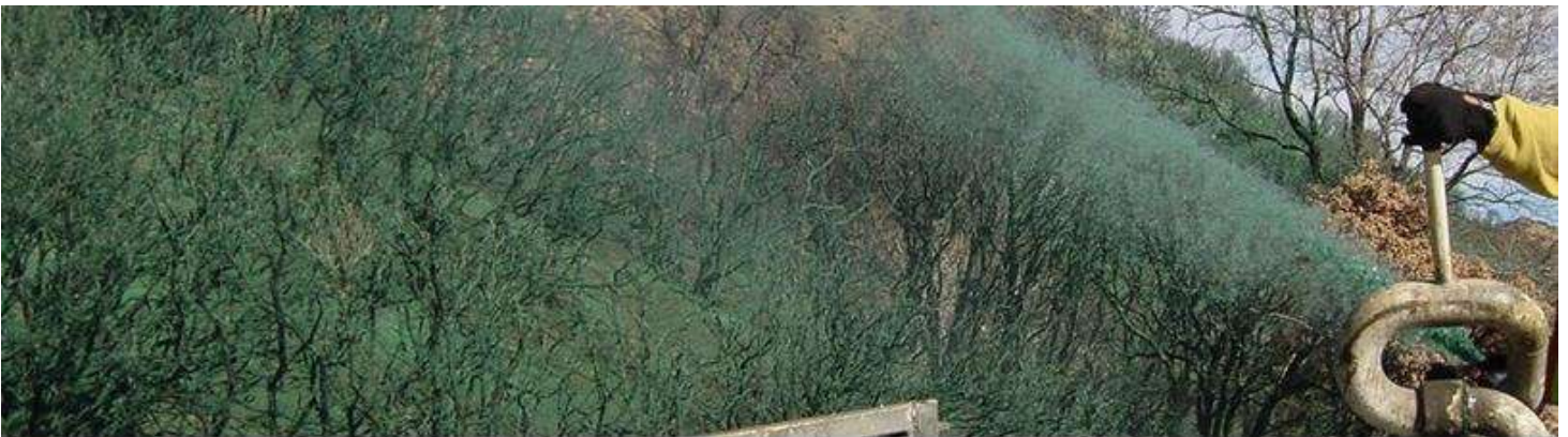
Hydroseeding a hillside
