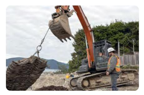
A blaster uses hand signals to communicate with a machine operator during placement of a blasting mat.
