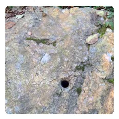
A bootleg or socket (an old blast hole) as seen from above
