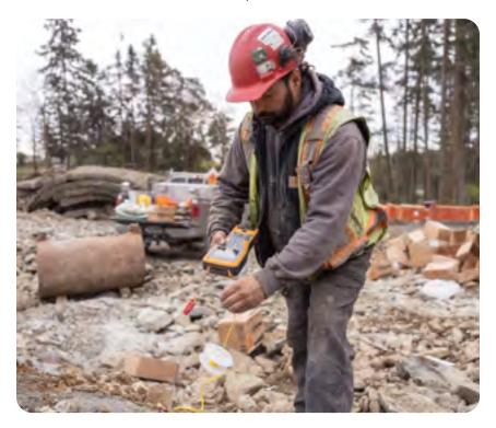
A worker programs an electronic detonator with a bench tester.
