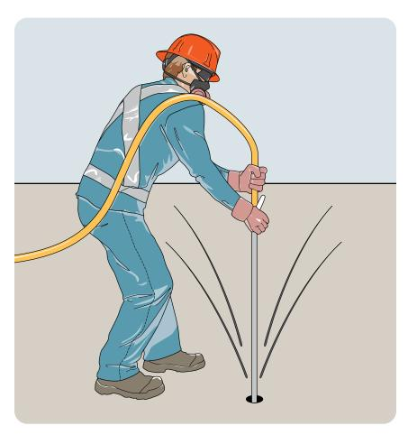
A worker uses a blow pipe to blow mud and rock out of a hole.
