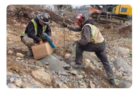
A worker compresses explosives into a blast hole with a tamping rod (loading pole).
