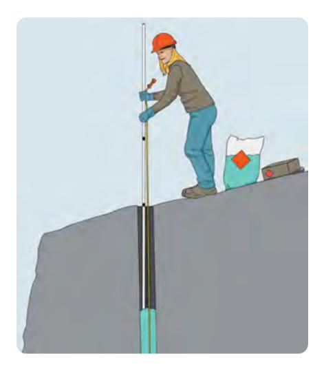
A worker controls the amount of explosives loaded in a hole by monitoring the collar length with a loading pole.
