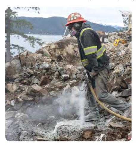
Hand-operated pneumatic rock drills expose workers to high levels of hand-arm vibration or whole-body vibration, depending on how the drill is handled. Other risk factors can increase the likelihood of injury from vibration, including the following:
