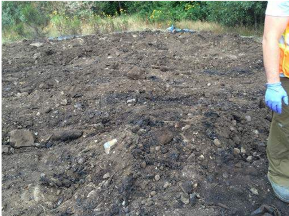
Soil contaminated with hydrocarbons may be contained in cells, or impermeable barrier lined pits, and treated over time with fertilizers and other catalysts to enhance the breakdown of the hydrocarbons. Photo credit: Chris Cole, RPF, P. Eng.
