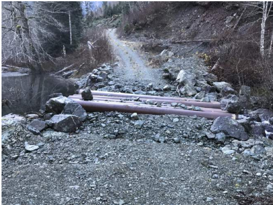
Example of a poorly designed and managed water crossing. Photo credit: Chris Cole RPF, P. Eng.
