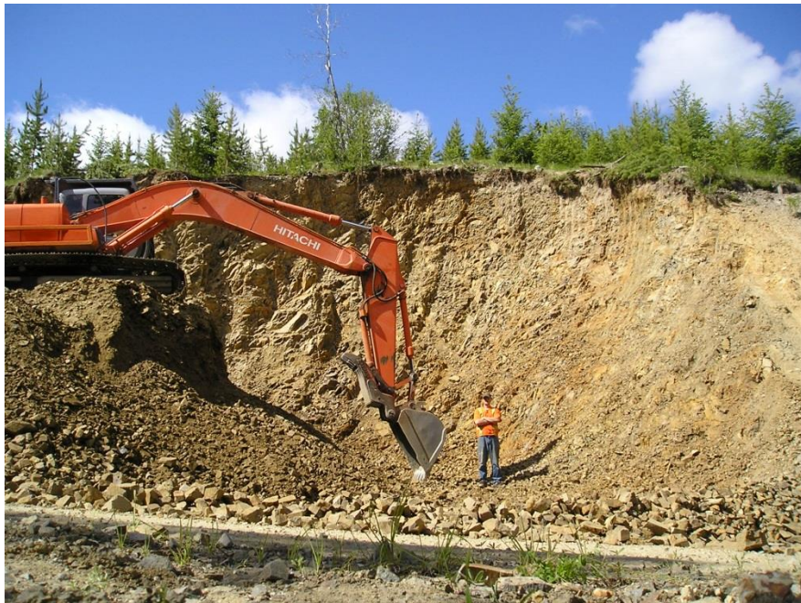
Borrow Pit Development for Road Re-surfacing Project. Source: Chris Cole, P. Eng.
