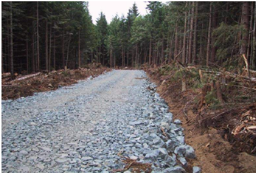
A new road is surfaced with shot rock in Haida Gwaii
