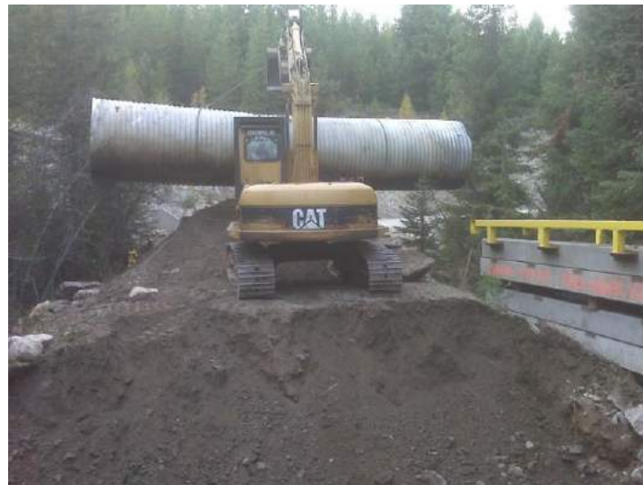
An old culvert is replaced with an open bottom concrete slab bridge a fish bearing creek near Kelowna, BC.
