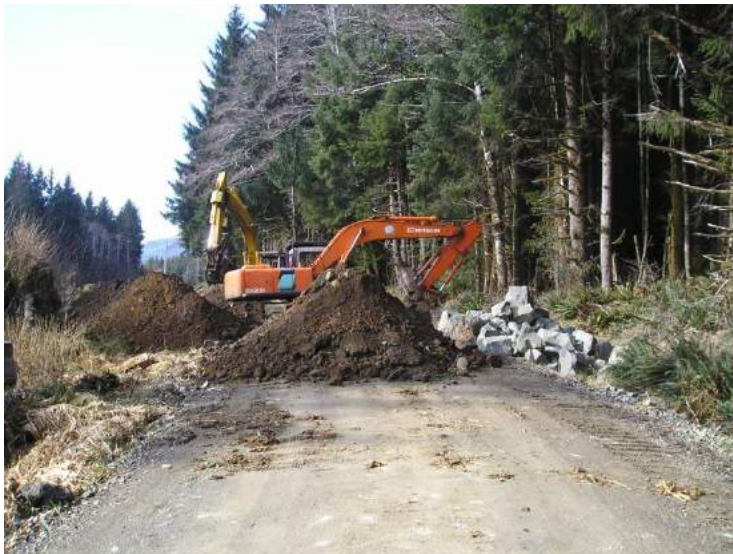
Road maintenance requiring the replacement of old culverts on Haida Gwaii
