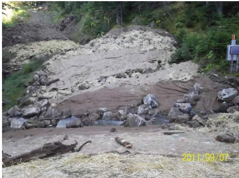
A stream crossing near Williams Lake, BC is deactivated in a community drinking water supply area. Extra measures were taken to minimize erosion, monitor water quality, and facilitate vegetation re-growth
