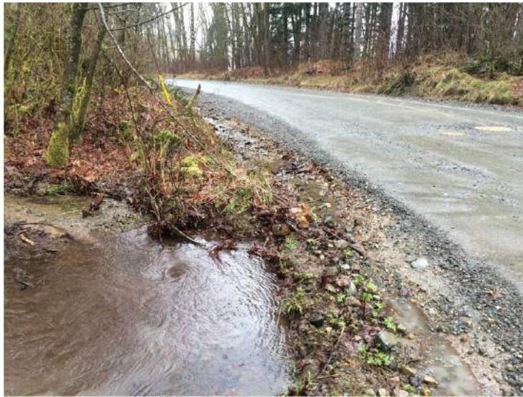
A plugged culvert prevents rain water to drain from a ditch near Lake Cowichan, BC
