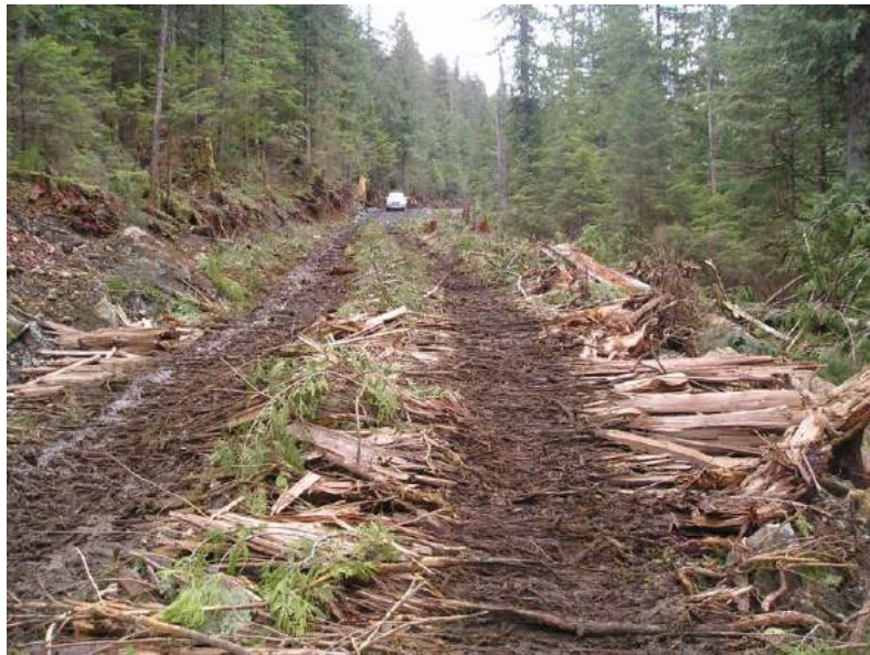
Puncheon used in the road subgrade on Haida Gwaii, BC coast
