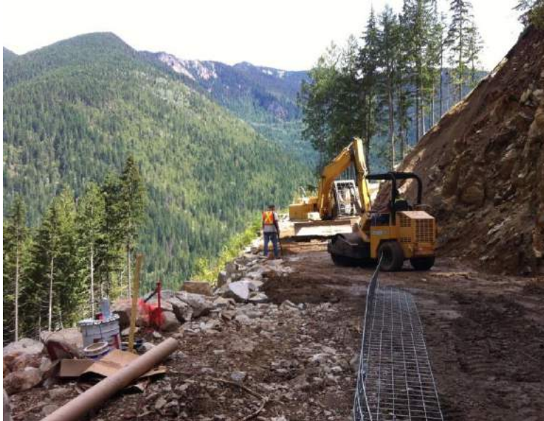
Road sub-grade is being prepared in steep terrain near Sicamous, BC
