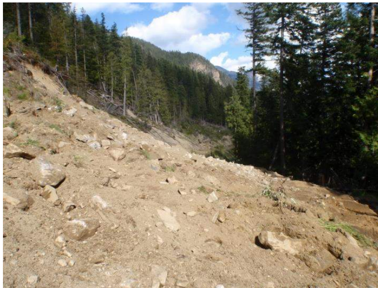
A road section is recontoured during deactivation near Quesnel Lake, BC
