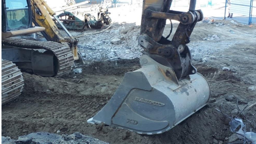
Bucket attachment on Excavator (Cambie and Broadway demolition site in Vancouver)
