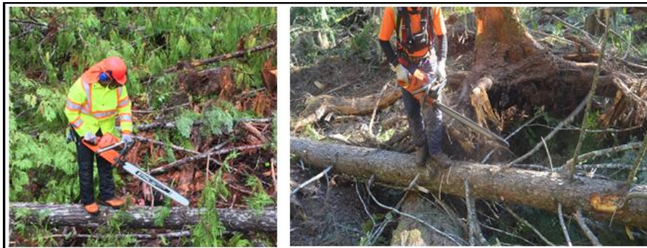
Figure 44: Safe limbing position while walking on the log
