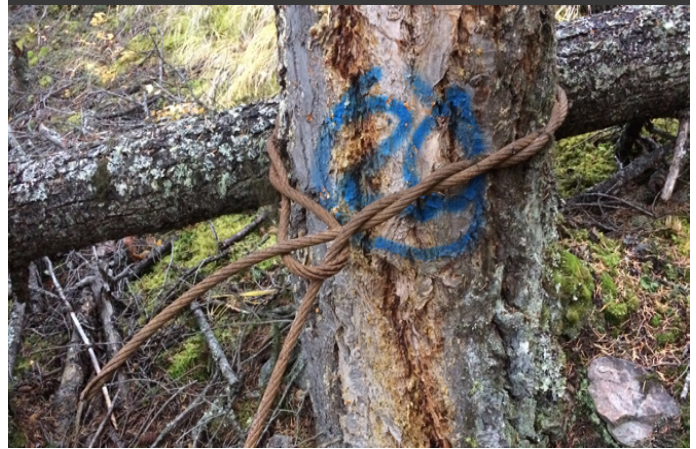
FIGURE 20. Pre-rigged anchor tree with extension strap
