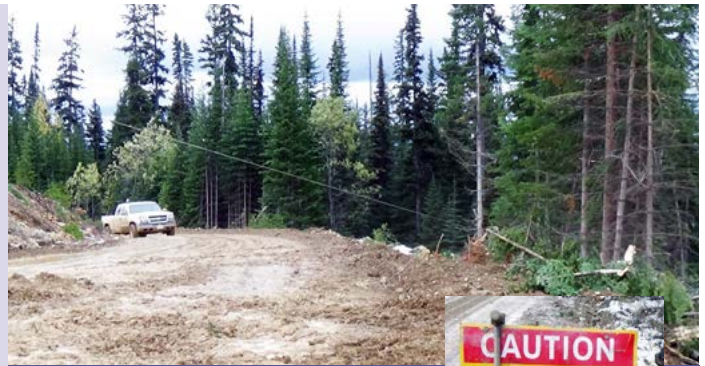
FIGURE 4. Identify any area where the cable crosses a road. Mark the cable with flagging tape to make it more visible.
