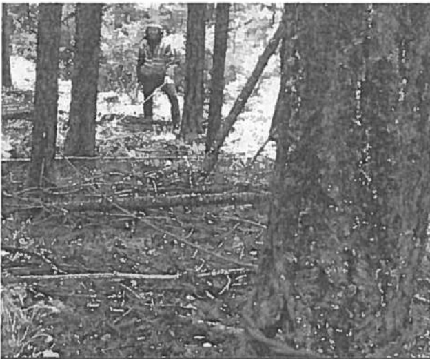
FIGURE 22. Multiple-tree anchor.
