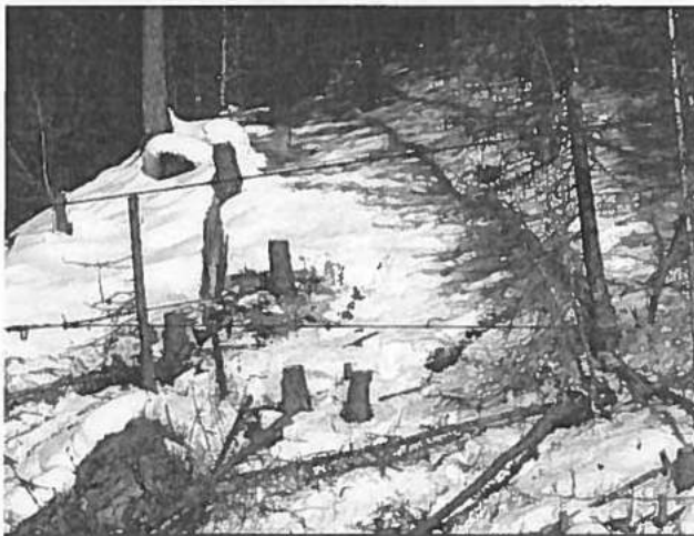
FIGURE 23. One-stump and one tree combined with an equalizer block for an anchor in small trees for a small cable-logging system.
