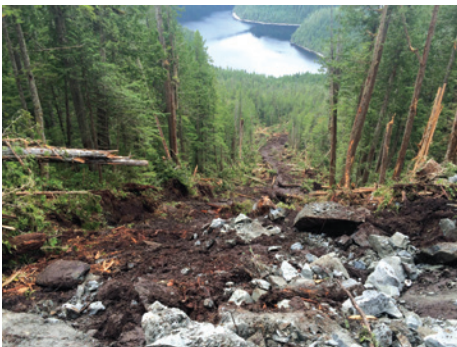
A sample of a road construction-initiated slide.
