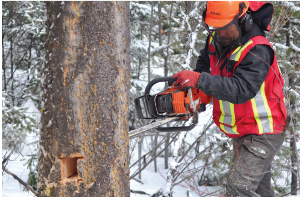
Prepping trees with the right cut (position and size) for the appropriate blasting material to control the blast and fall of the tree as intended, and documenting everything.
