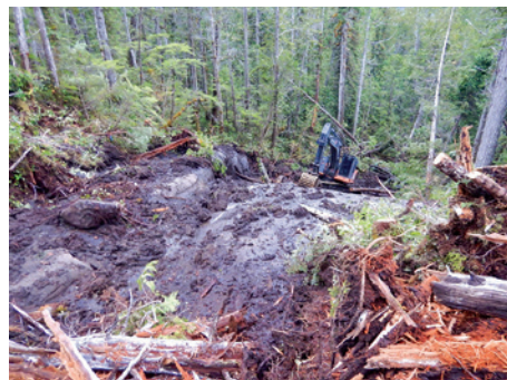
Excavator in a construction initiated slide.
