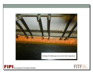
Sealing cracks, for example of cableways though walls, prevents dust migration from one area another, or to prevent dust from accumulating in wall and ceiling cavities
