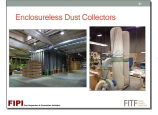
On this slide, we have two examples of enclosureless dust collectors.
