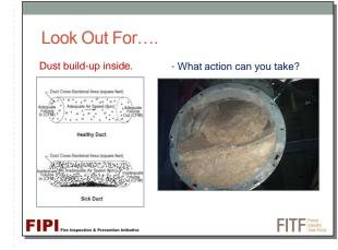
When you observe dust buildup inside dust transport ductwork, it means the duct work is not designed properly or the transport velocity is too low allowing the dust to settle somewhere inside the duct work.
