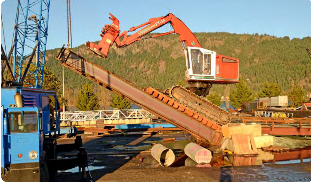
FPIinnovations tests equipment to help shape better performance and safety outcomes.
