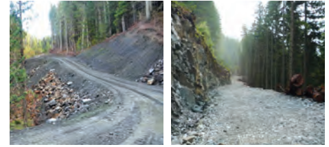
Three examples of good road construction on steep slope, demonstrating a good plan and working the plan with qualified professionals to ensure stable, safe forestry roads for industrial and public use.
