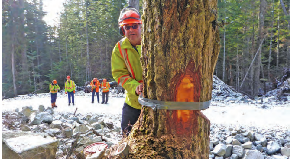
Glenn Hestnes, BC Forest Safety Council falling safety advisor, prepares a tree along road right of way for blasting.
