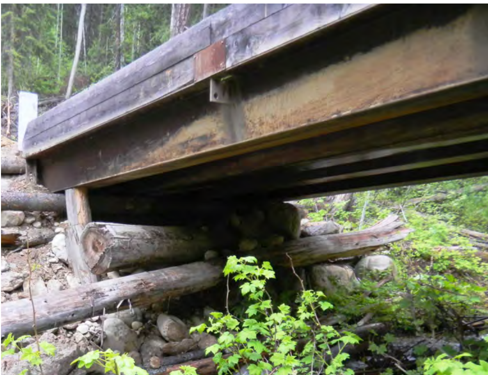
Top: Example of a safe bridge. Bottom: Example of an unsafe bridge. Photos provided by the Forest Practices Board.
