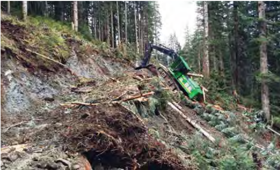
A sample of a construction initiated slide near Terrace, BC. Photo courtesy of Brinkman Forest Ltd.
