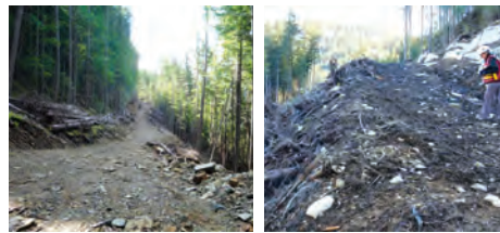
Two examples of poor road construction on steep slopes (above). The one on the right is on the coast and "the road" was constructed out of slash.
