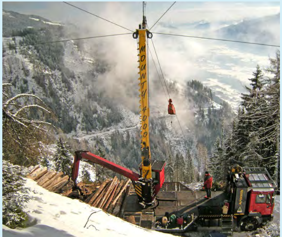
A cable-yarding operation in Austria. The owner came out to British Columbia to learn more about our forest safety systems and take the BC Forest Safety Council small employer training course.
