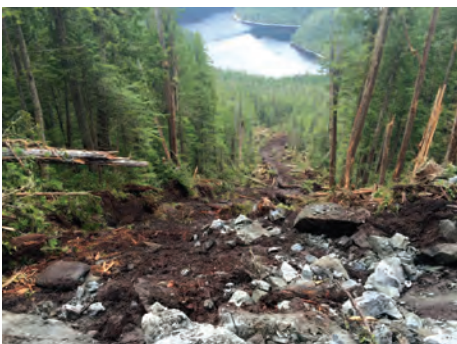
An example of a construction initiated slide.
