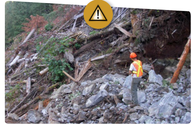
Full bench endhaul section under construction. Unless controlled, hazardous roadside debris will be present below the centerline.
