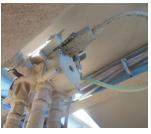
Do not overtighten wires onto air hoses with tie wraps; this may cause wire pinching as hoses expand.
